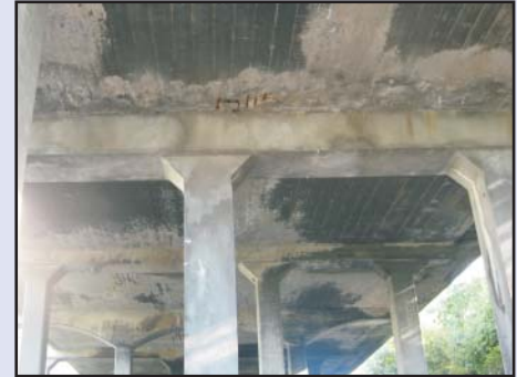
Broadway bridge near 37th St. South
